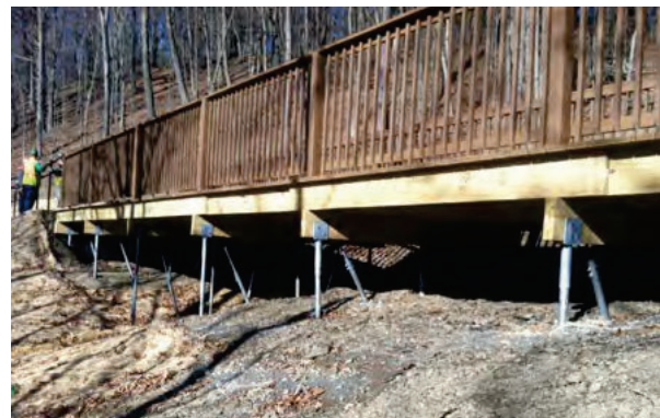
Figure 1.30 Boardwalk supported on vertical and battered helical piles
