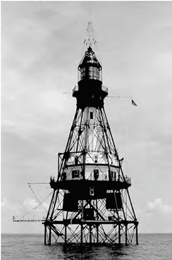
Figure 1.1 Lighthouse supported by screw (helical) pile foundations
