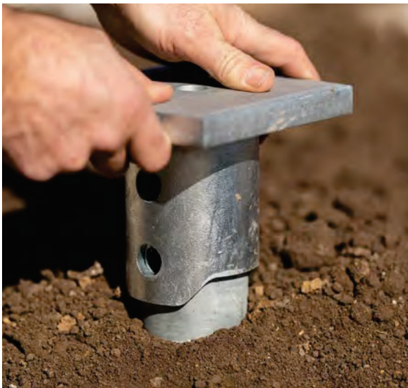
Figure 1.76 Install new construction bracket
