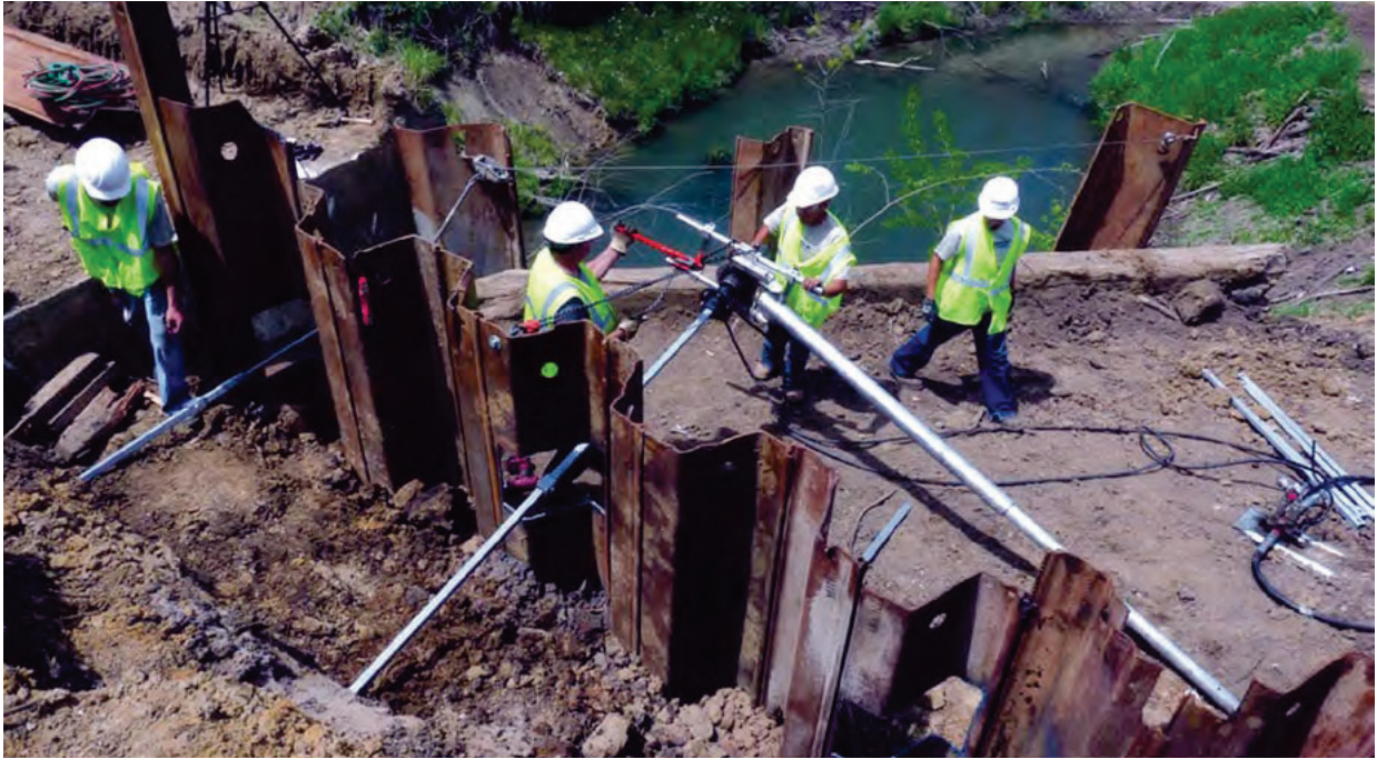
Figure 1.5 Helical tieback installation with hand-held equipment
