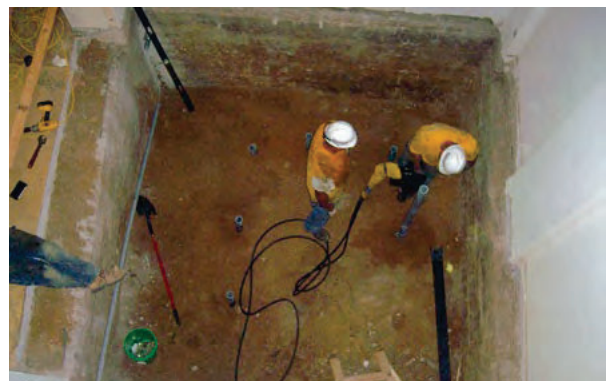
Figure 1.34 Helical piles installed with hand-held equipment to support new elevator within existing school
