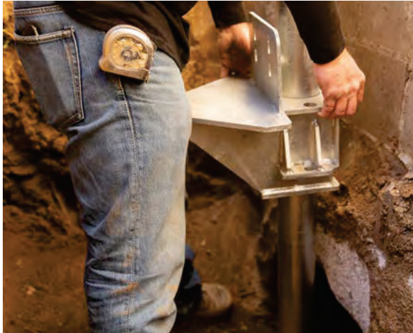
Figure 1.80 Lower assembly over pile shaft
