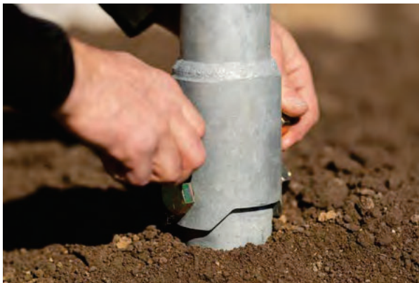
Figure 1.75 Install coupler bolts
