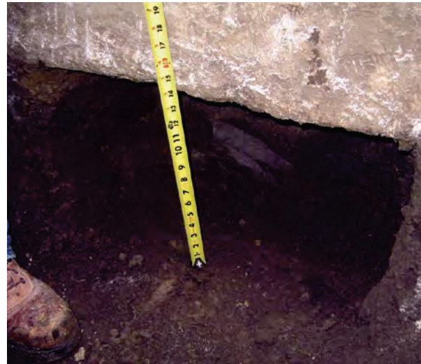
Figure 1.77 Excavation at bracket
