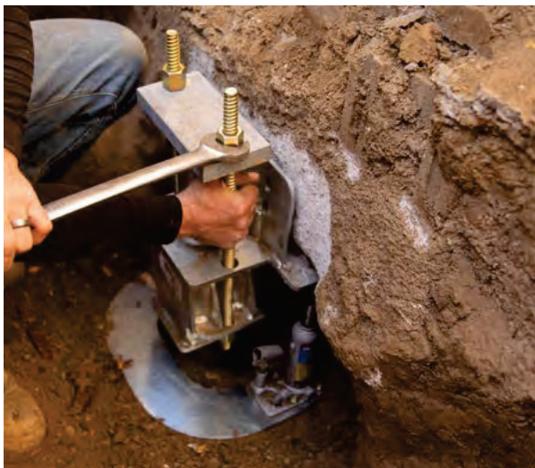
Figure 1.82 Install cap plate and rods
