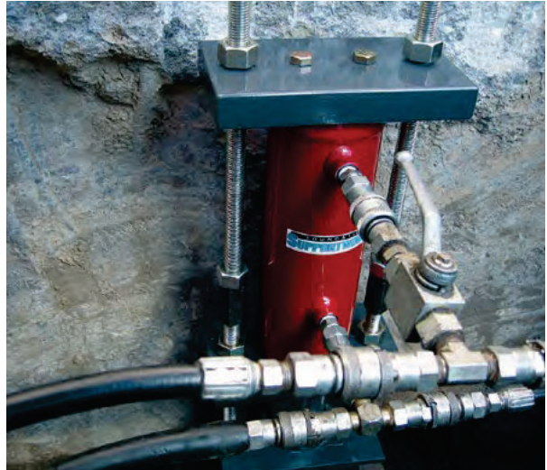
Figure 1.83 Set hydraulic lift cylinders
