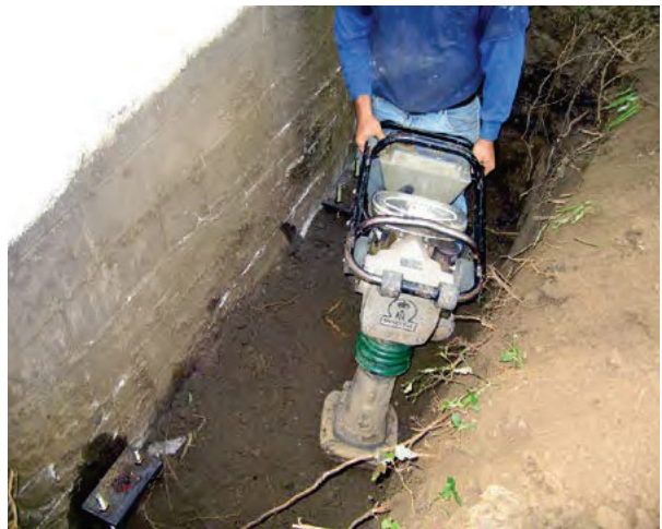
Figure 1.84 Backfill and compact soil
