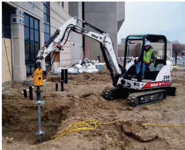
Figure 1.3 New construction helical pile installation
